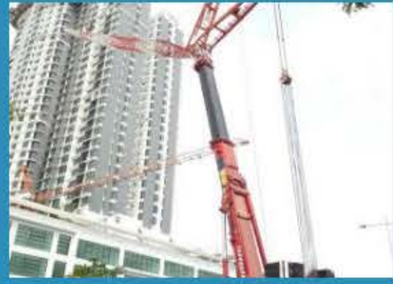
Dismantle Tower Crane
