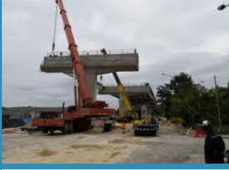
DASH (Damansara - Shah Alam Elevated Expressway)
