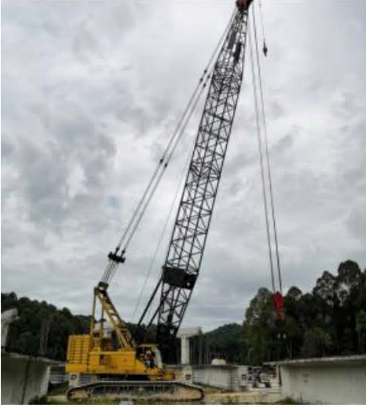
250T Crawler Crane
